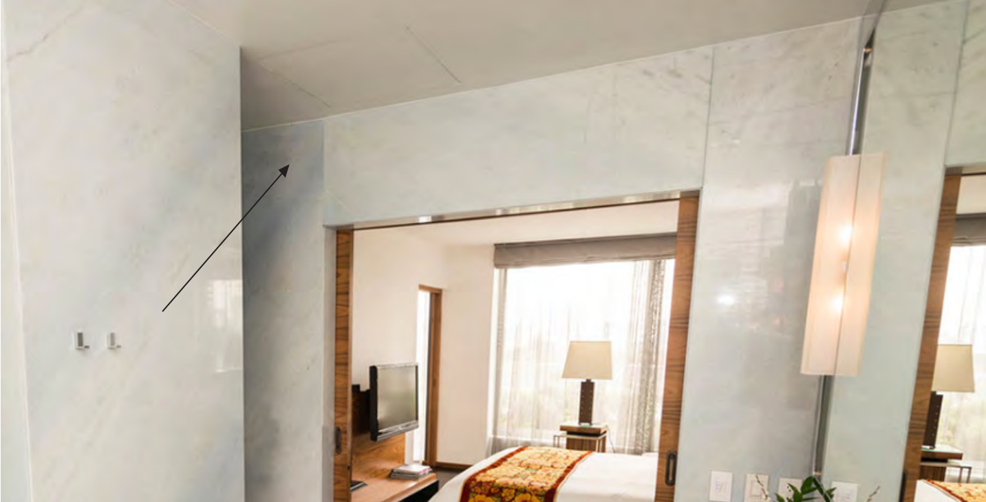
Ceiling Installation in Las Alcobas Resort - Mexico City
